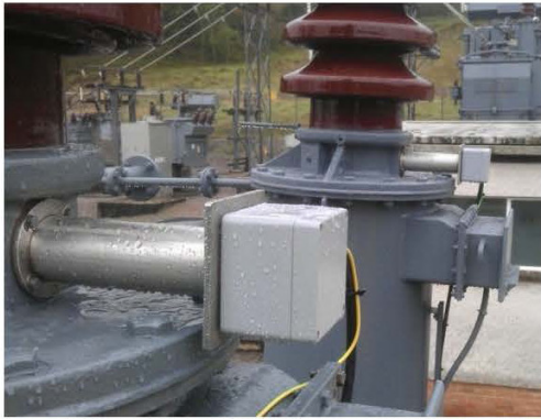
Fig 10 Adapters Fitted to the Bushing Taps to Allow TW Fault Location
