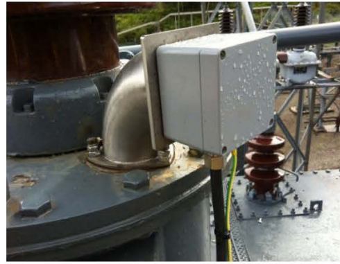
Fig 10 Adapters Fitted to the Bushing Taps to Allow TW Fault Location
